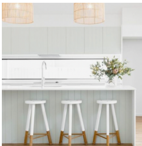
VJ finish to back of island bench
